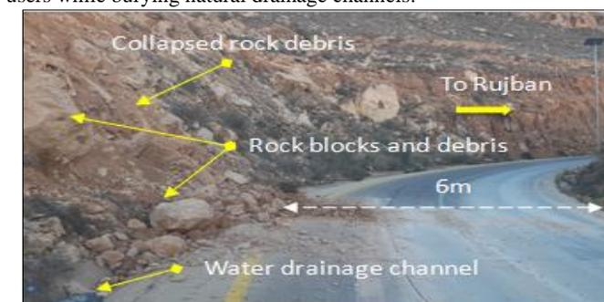
**Fig. 2:** Rock Debris Collapse at the Study Area Site
