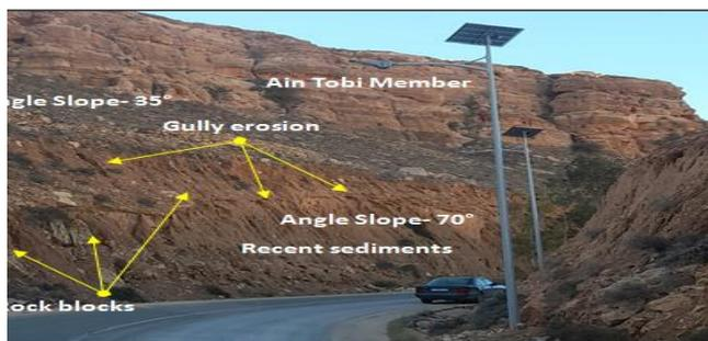
**Fig. 1:** A section of Rujban Mountain Road The collapse. led to road closure, and the debris was removed by road users while burying natural drainage channels.
