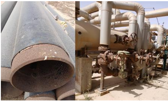
Fig. 6: Kinds of anti-corrosion coating for pipeline.
