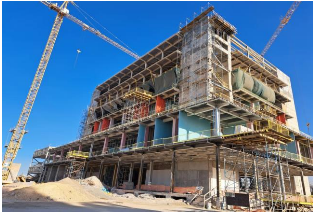
Figure (1) : Existing steel structure building (5 TH and 6 th floor constructed recently based on designer decision).
