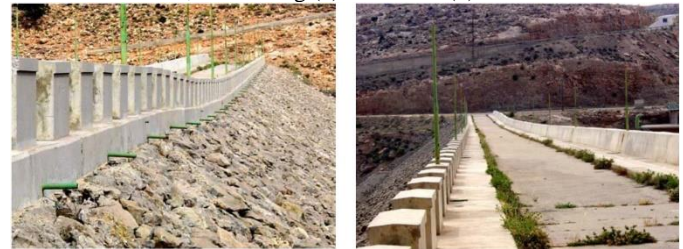
Fig. (3). Abu Mansour Dam vertical deformation as seen from the right abutment (A) and horizontal deformation as seen from the left abutment (B) after [11].
