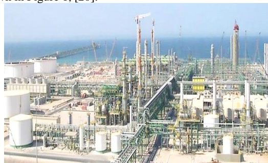
Fig. 1: The Mellitah gas plant [20].
