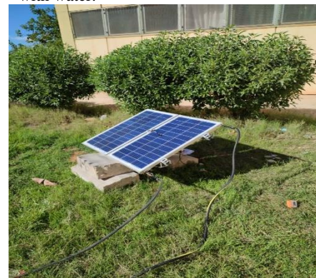
Figure 6 panels, one with cooling and the other without cooling.
