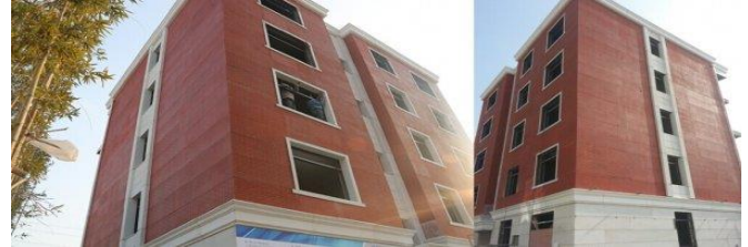
Fig. 14: The world's highest 3DP structure with five stories consisting of assembled structural elements [40]
