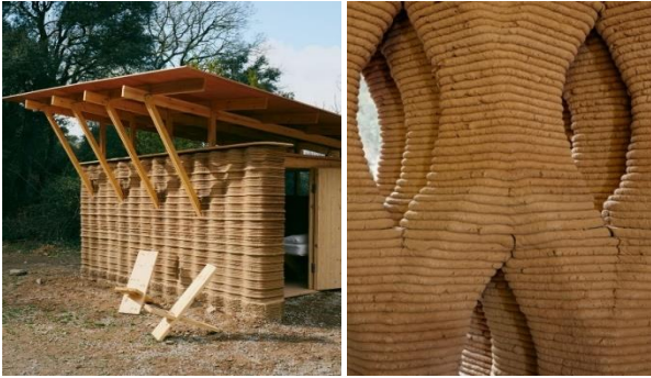
Fig. 11: The first structure TOVA in Spain was created by 3DP and Earth [36]
