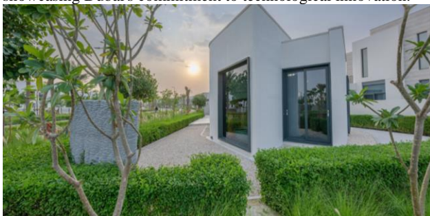
Fig. 7: The first 3D-printed villa with smart house technologies - Dubai [32]
