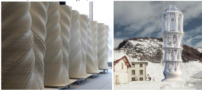
Fig. 6: The tallest 3DP structure -Tor Alva- to April 2024 [31]
