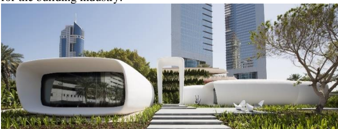
Fig. 13: The world's first fully functional and permanently occupied '3DP' building (The Office of the Future) [39].
